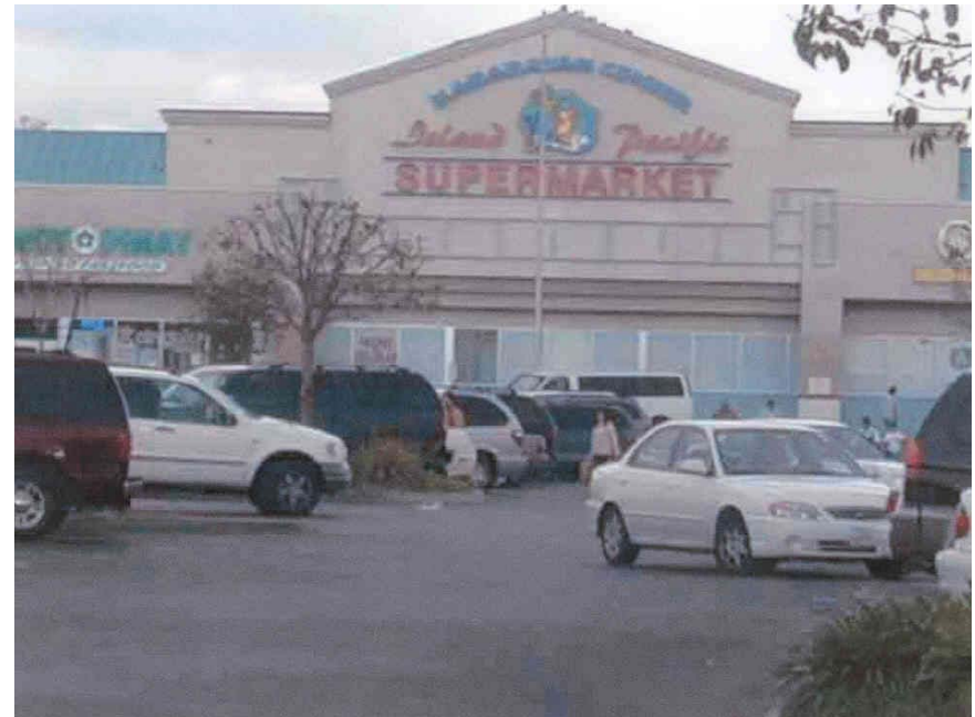
This is an opportunity for a pedestrian walkway connecting commercial facilities on both sides of Van Nuys Boulevard.
