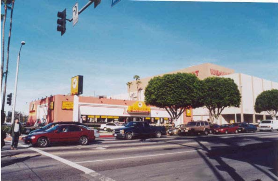
Existing commercial area at the northwest corner of Van Nuys and Roscoe Boulevard.
